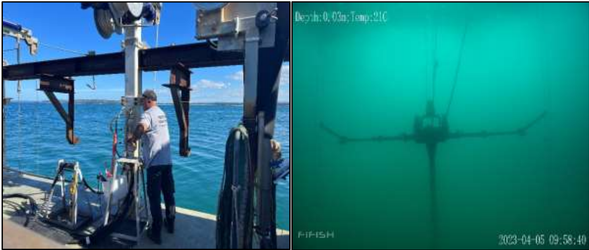
Figure 4:SCM crew deploying anchors using Screw-in Anchor Technology by Marine Flex Ltd (Source: SCM 2023)
